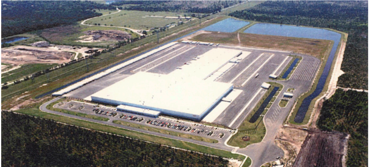
Figure CS3-13. BJ's Wholesale Club warehouse, cross-dock, and freight yard near Jacksonville, Florida. Cowan Systems is co-located at this complex. (top) BJ's Wholesale Club locations in south Florida (bottom).
