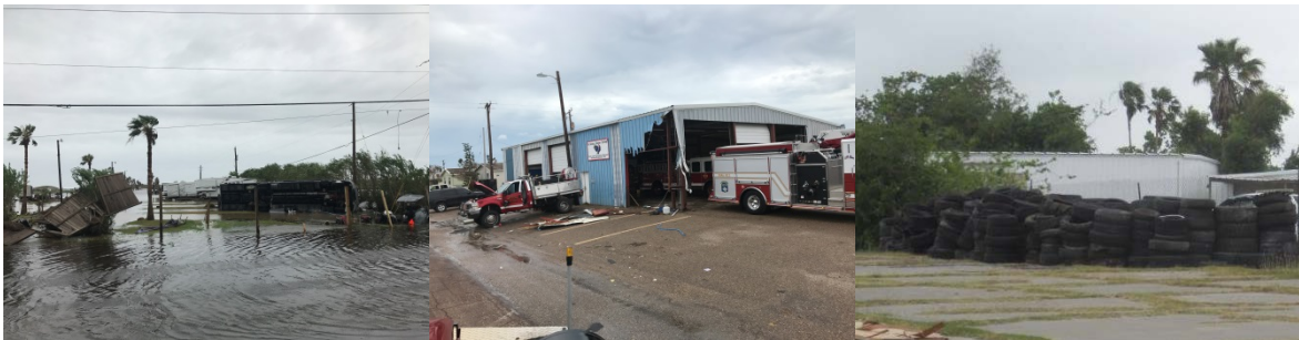
Figure 5. CS4-4. Water pooled in Port Aransas is a breeding ground for mosquitoes (left). The Port Aransas Fire Department roof is mostly intact, but the building sustained damage (center). Used tires in Aransas Pass (right).
