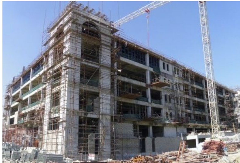
Construction site of the Ministry of Defense in Afghanistan (NATO Training Mission Afghanistan photo/photographer unknown).
