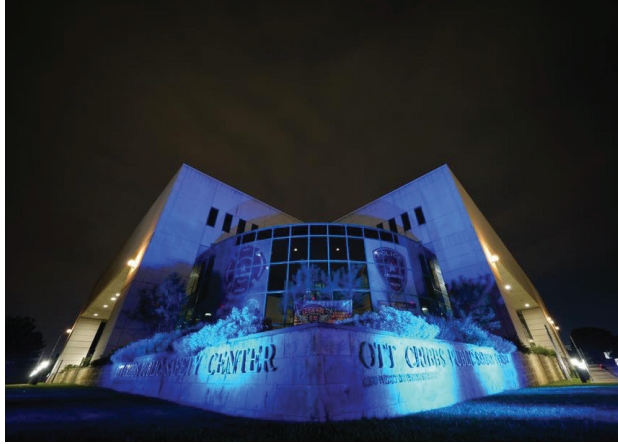
Ott Cribbs Public Safety Building, Arlington, Texas
